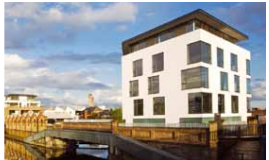
Westbourne Grove Canal Building, London
